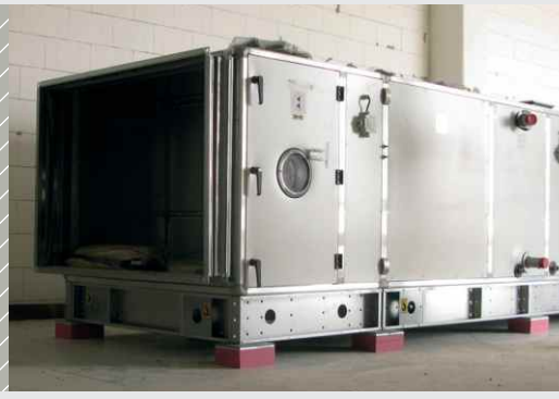
Vibration protection for air-conditioning system
