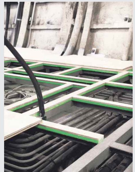
Decoupling of yacht flooring
