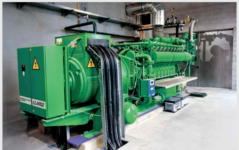
Machine foundation bearings
