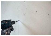
8 The tongue and groove of the panels are screwed together at an interval of 15 cm.
