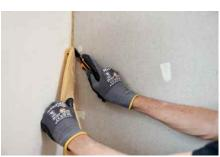
Cut the protruding lateral insulation strip and seal off the edge joint using acoustic sealant.
