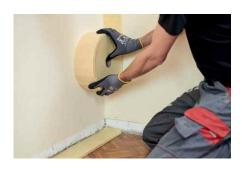
Fully line all adjacent components such as floors, ceilings and lateral walls with a double layer of edge insulation strip. Use acoustic sealant to secure.
