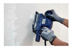
The sound control system has now been installed and the surfaces are ready to be trowelfinished, sanded and painted.
