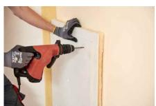
Place the panels in position on the wall. Drill holes for the fastenings into the supporting wall through pre-fabricated anchor points.
