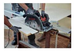
4 Start installing from the bottom left. Cut the tongue of the first panel on the short and long sides. Only cut the tongue on the long side of the panels above.
