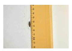
The overhang should be at least 25 cm long. In order to avoid sound bridges, check the thread reach of the attachment points again before continuing to install the drywall.
