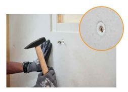
6 Then insert and screw in the screws, washers and dowel plugs provided.
