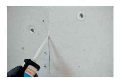
Sand the transitions and fill the joints with acoustic sealant. Then you can easily screw a standard plasterboard to the underlying sound control panel.
