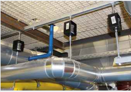
Pipework suspension with Isotop SD/Z
