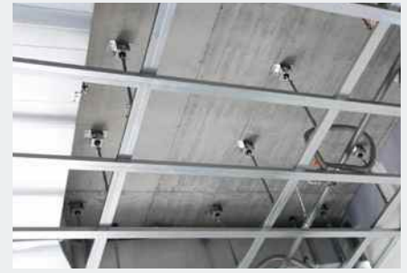
Ceiling hanger Isotop MSN/Z-LC
