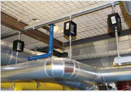
Pipework suspension with Isotop SD/Z
