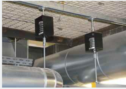
Decoupled pipes with Isotop SD/Z
