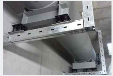
Bearing of duct silencer
