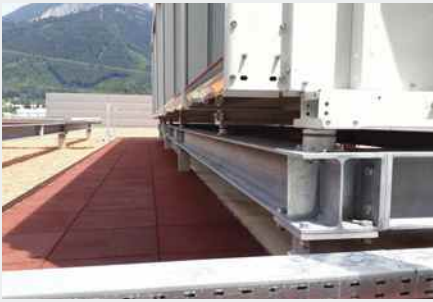
Recooler with Isotop DZE versus high wind loads
