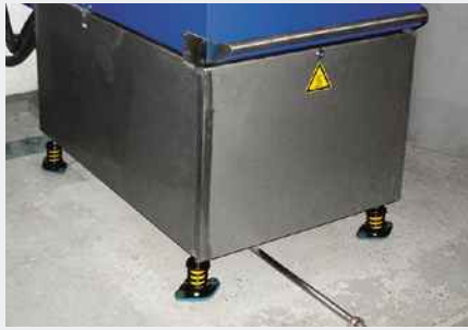
Small combined heat and power plant
