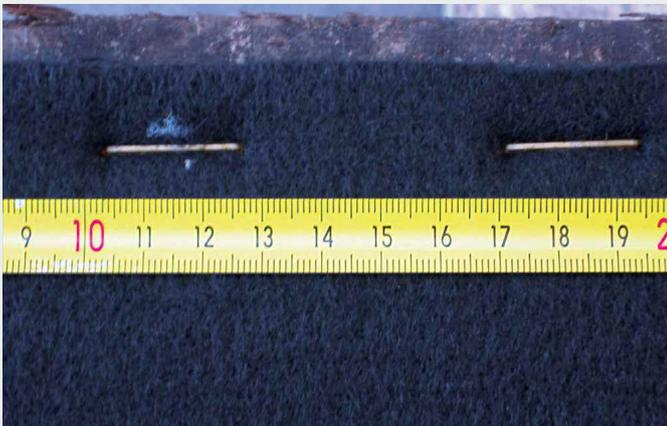
The staples should be placed with a spacing of 4 to 5 cm between each other.
