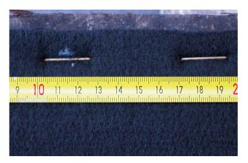
The staples should be placed with a spacing of 4 to 5 cm between each other.
