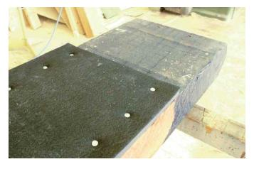
Driving the nails into the material has to be performed very carefully to ensure that the resilient layer is completely attached to the timber sleeper and not penetrated and damaged by the nails.
