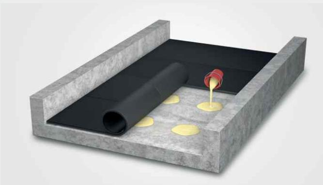
Firstly one half of the UBM is folded from one sidewall to the other one to uncover half of the track bed. After this half is glued, the same steps are repeated for the other half.
