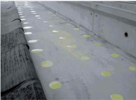
Avoiding displacement during ballasting, the mats can be glued to the sub-base. The adhesion must be longitudinally along the area of the track position and at the transition to the sidewall mats (about 100 mm at the edges).
