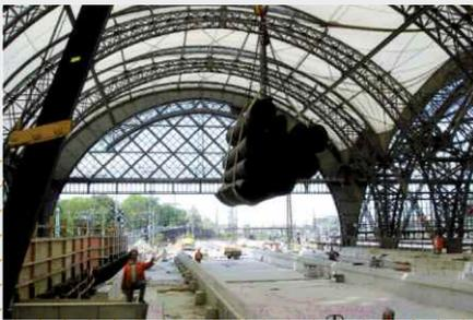
**G**etzner ballast mats corresponding to the type, their thickness and weight are delivered in rolls and therefore very easy to handle. The side of the mats facing the ballast is protected by a geo-textile. This geo-textile has practically two functions - as a protective layer against ballast-grain penetration of the spring layer as well as a load-distribution layer throughout the load bearing area.
