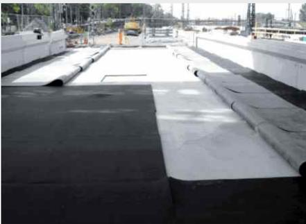
The connection of the mats will be made by a getzner-specific welding machine and a strip of 10 cm which covers the slit between the USM. Alternative: the strip which covers the slit can also be glued by a PU-Adhesive. Subsequently to the ballast mats the sidewall mats are installed. They are mounted onto the ballast mats. To keep the overall calculated height, the thickness of the ballast mats is subtracted from the actual sidewall mats.
