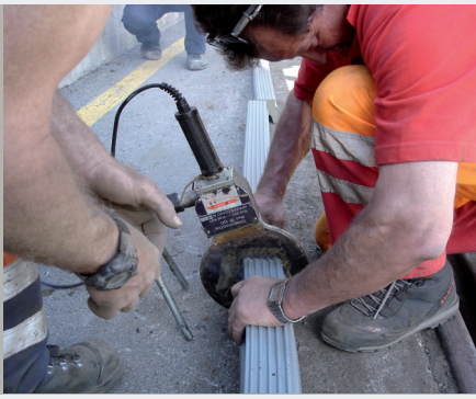
Welding the groove filler profiles together
