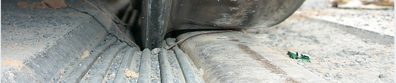
Installed Sylomer® Rail Groove Fillers with wheel flange
