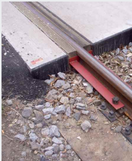
Installation in slab track
