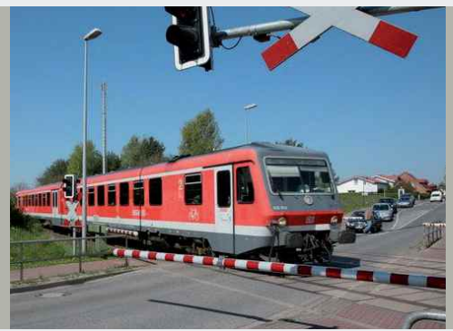
Level crossing with Sylomer® rail groove fillers
