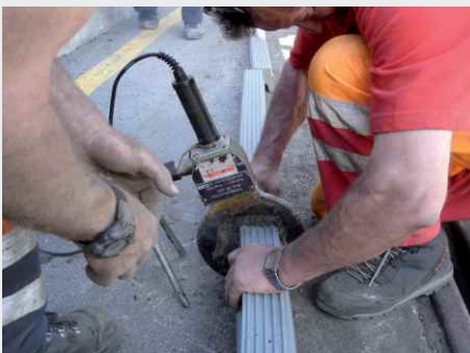
Welding the groove filler profiles together
