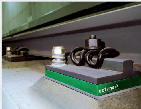
Differences in track stiffness caused by components such as the crossing frog in turnouts lead to dynamic shocks during the passage of trains. This results in additional stresses on the entire track superstructure. Grooved baseplates of various sizes require special attention in elastic mounting systems using baseplate pads.
