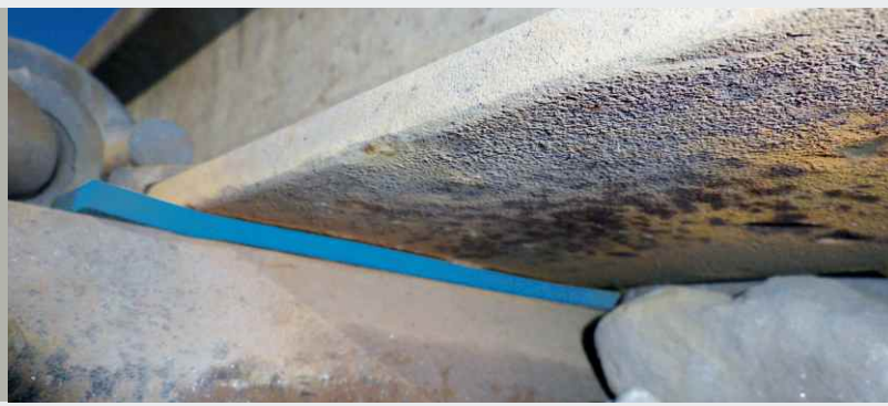
Installed rail pad
