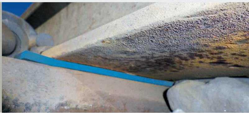
Installed rail pad
