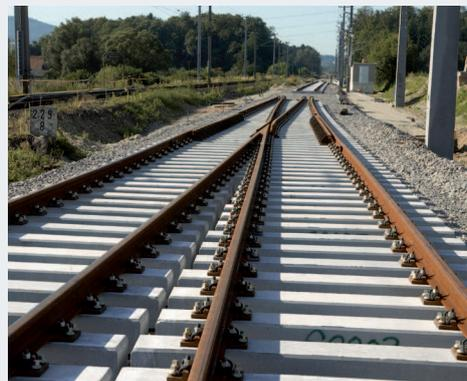
**T**he stiffness of the bedding varies in turnouts on ballasted track due to the various lengths of the sleepers and components which increase track stiffness such as the crossing frog, check rails and wing rails. The resulting dynamic loads caused by passing trains increase the LCC, and reduce the level of comfort, and moreover the vibrations caused can be transmitted into neighbouring structures.
