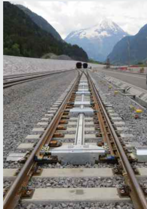
Turnout tunnel portal
