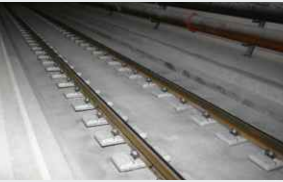
Slab track with LVT system
