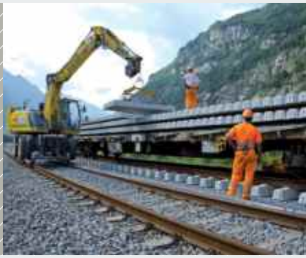
Lines feeding into the tunnel with ballast superstructure
