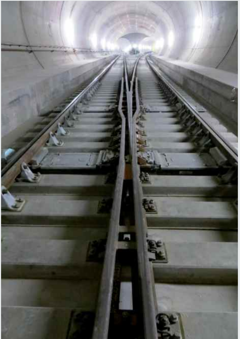
Slab track turnout
