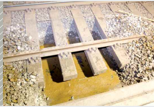
Exposed under ballast mat
