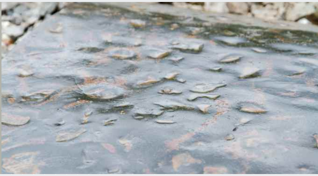
Imprints of the track ballast on the under ballast mats
