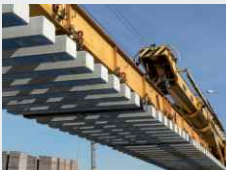
Installation train with switch padding
