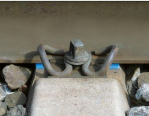
Installation of rail pads Unzmarkt Scheiffling, Austria
