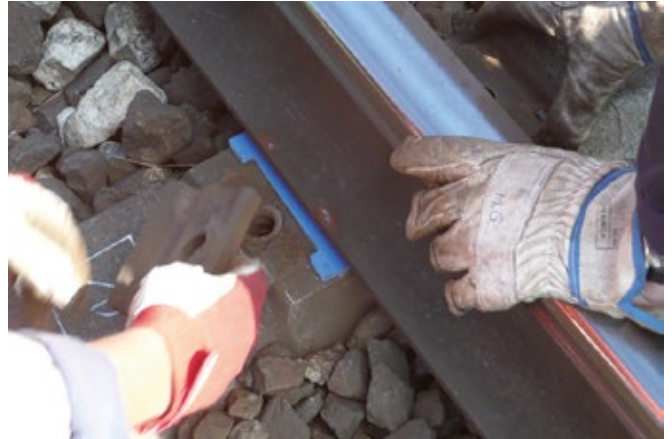
Installation of rail pads
