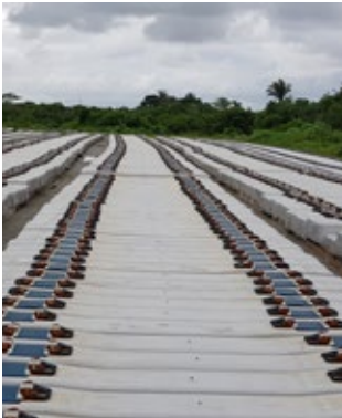
Installation of rail pads Vale Cavan, Brazil
