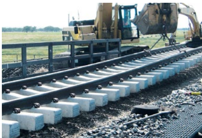
Installation of under ballast mats on a section of Union Pacific track in the USA
