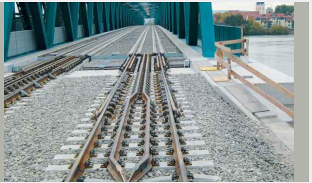
Transition area on a steel bridge
