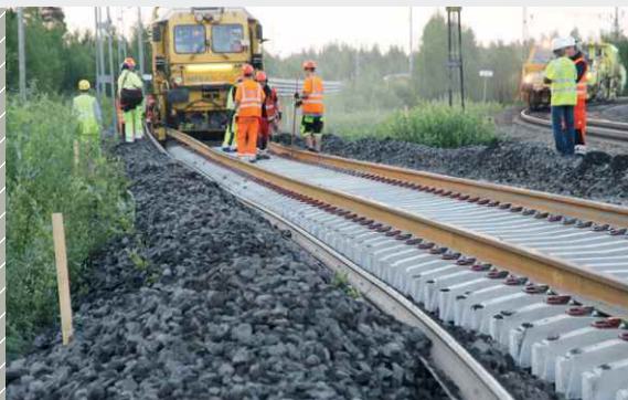
Installation of padded sleepers on the Malmaban route
