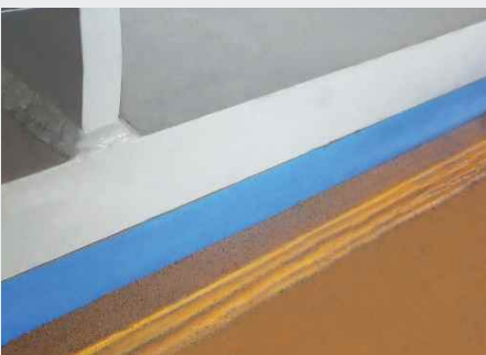
Elastic bearing of a turbine
