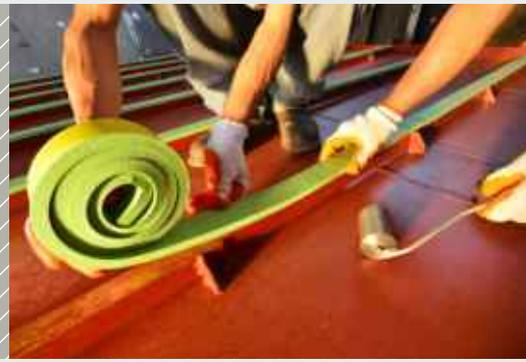
Installing the vibration bearing using Sylomer® strips
