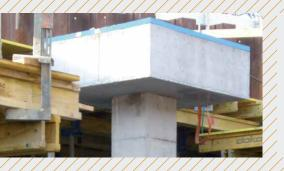
A high-resilient bearing from Getzner Werkstoffe can support a comparable load of roughly 600 tons on an area of one square meter.
