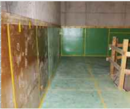
Full-surface foundation bearing on Sylomer®
