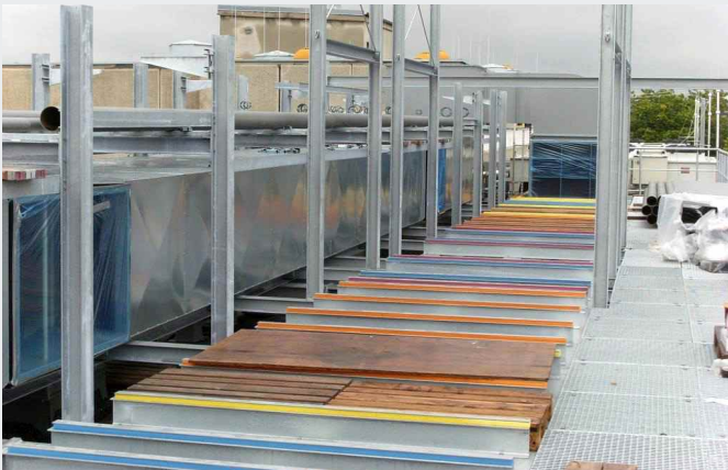
Strip bearing prepared for a rooftop ventilation unit
