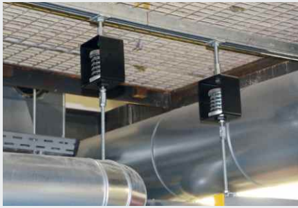
Decoupled pipes with Isotop SD/Z
