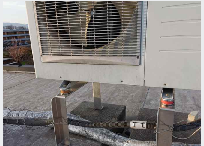
Heat pump bearing with Isotop Compact
