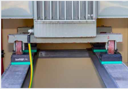
Vibration decoupled bearing of a distribution transformer
