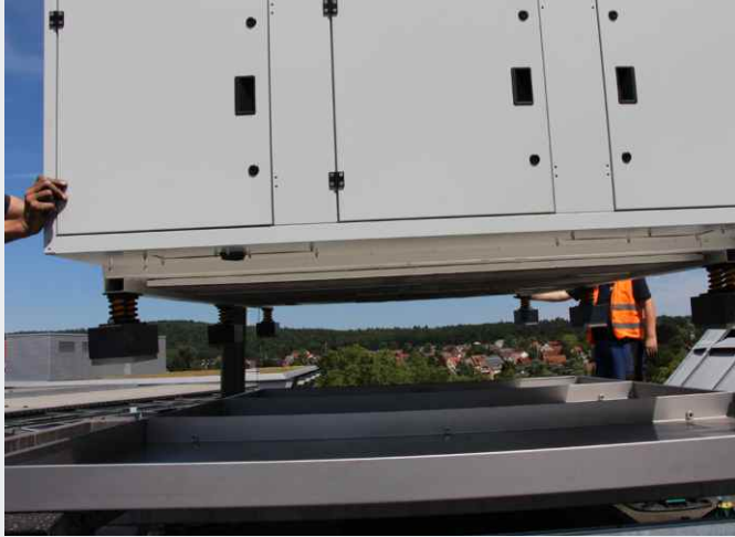
Unit installation with pre-mounted Isotop DT
