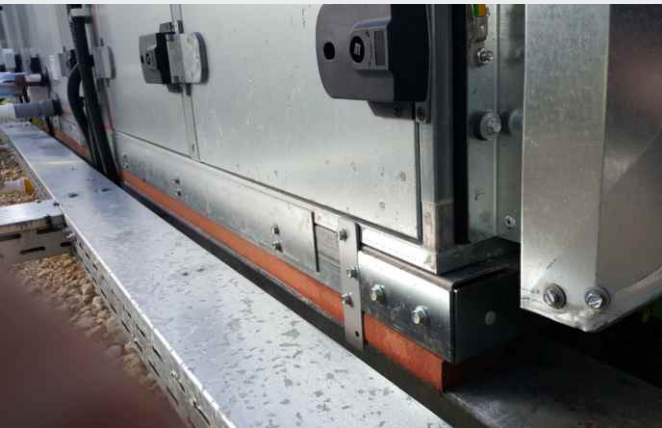
Strip bearing for ventilation and air-conditioning unit (HVAC)
