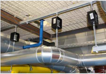
Pipework suspension with Isotop SD/Z
