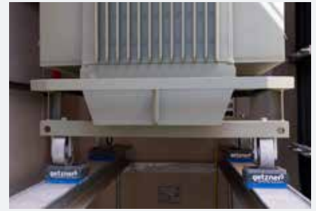
Vibration decoupled bearing of a distribution transformer
