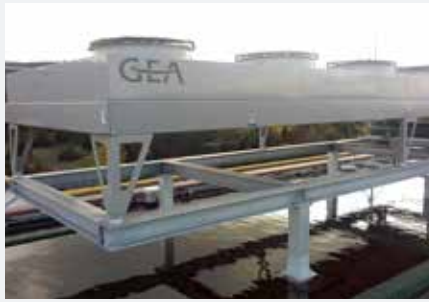
Recoiler with Isotop® DZE to counter very high wind loads
