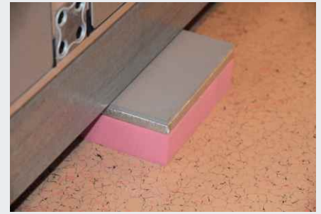
Air conditioning unit on Isotop SE pro
