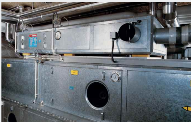
Decoupled air handling unit module
