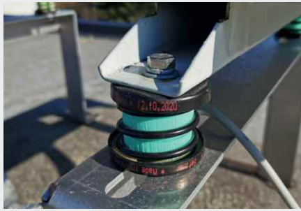
Monoblock heat pump with Isotop DMSN
