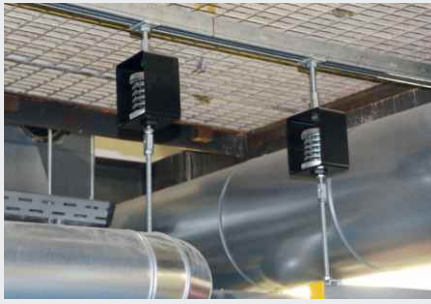
Decoupled pipes with Isotop SD/Z
