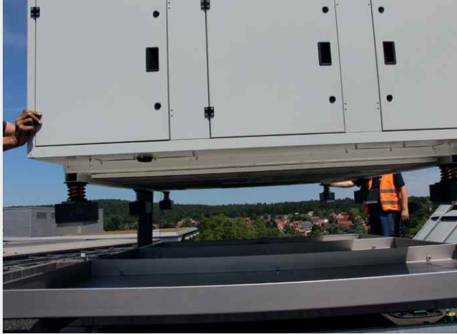
Unit installation with pre-mounted Isotop DT
