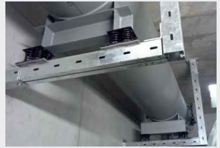
Bearing of duct silencer
