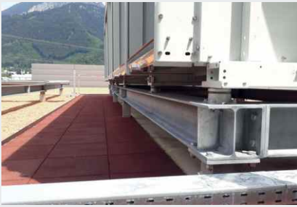
Recoiler with Isotop DZE versus high wind loads
