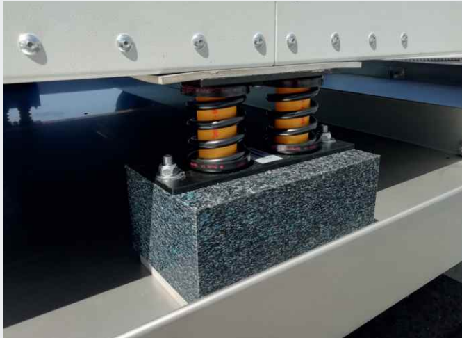
Air conditioning unit with Isotop DT and Isotop DSD-BL2 (not included in the scope of supply)
