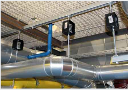
Pipework suspension with Isotop SD/Z
