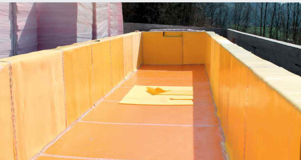
Full-surface installation of Sylomer® at the Villa Aurea
