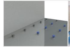
4a) Place the floor blocks by type according to the installation plan.
