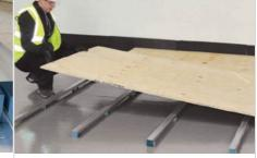
5) Laying the lost formwork (OSB - panels).
