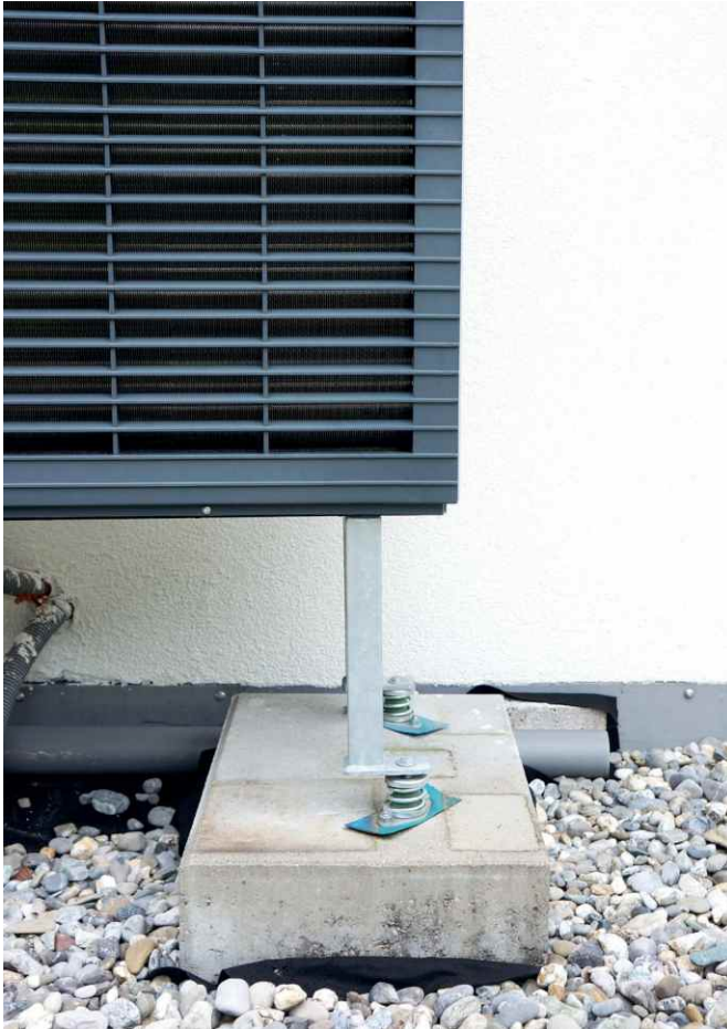
Bearing of an outdoor unit on the floor (footing) using Isotop® MSN elements
