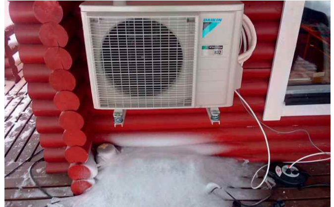
Bearing of a suspended outdoor unit using Isotop® MSN elements
