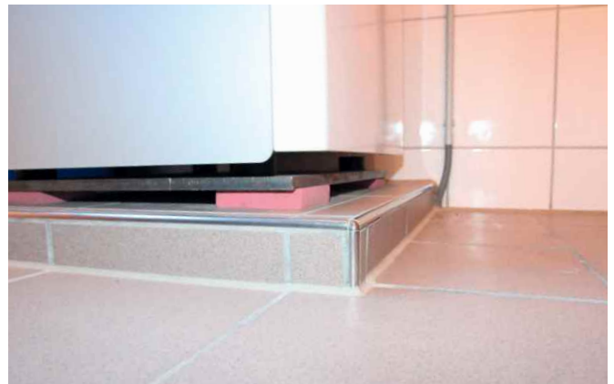
Decoupling of an indoor unit using Sylomer® point bearings
