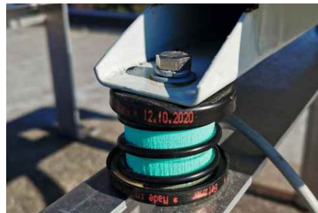
Bearing of a heat pump with Isotop® DMSN
