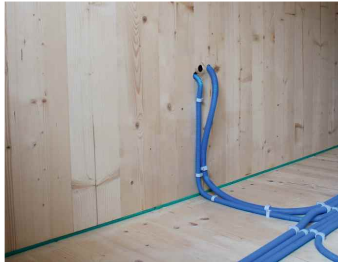
Sylodyn® strip bearing: Decouples flanking sound and offers more privacy in interior spaces
