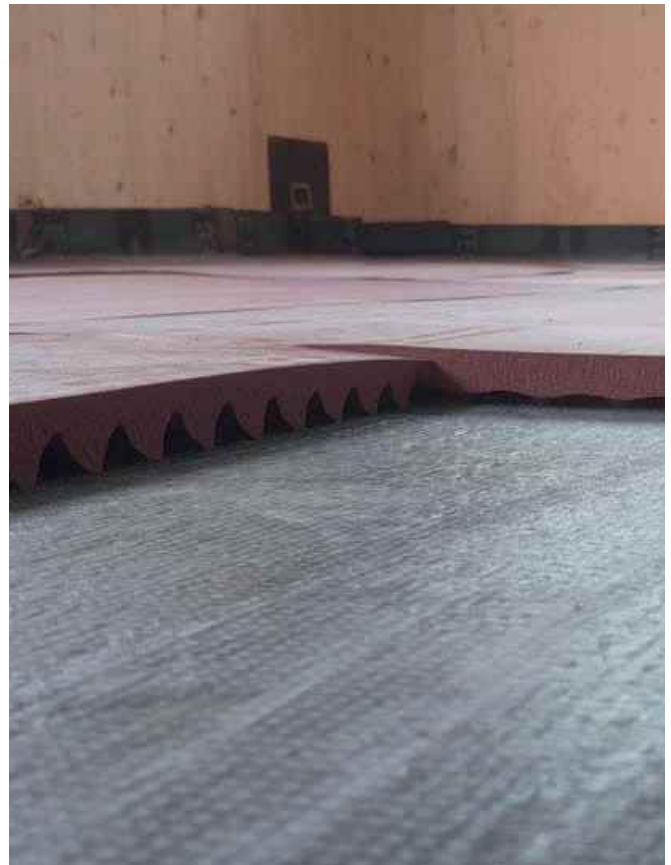
AFM35: Sustainable isolation with high acoustic effectiveness
