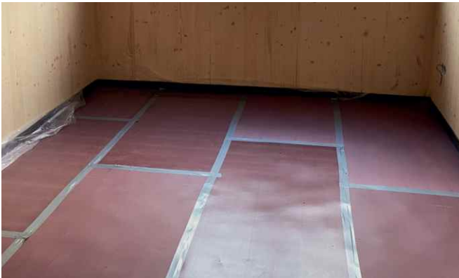
AFM35: Low-frequency impact sound insulation for optimum vibration protection
