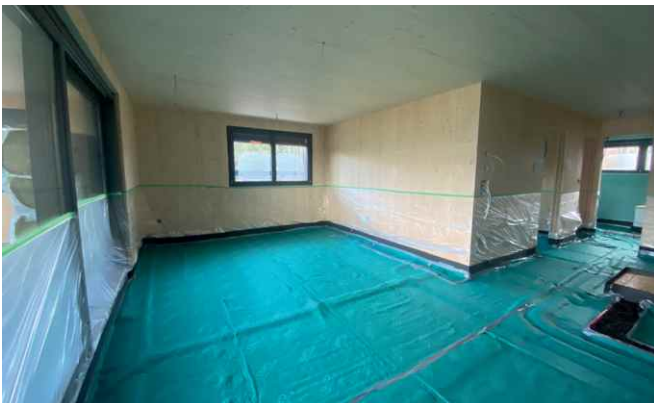
GREI: Recycled EPDM/SBR layer to reduce impact noise
