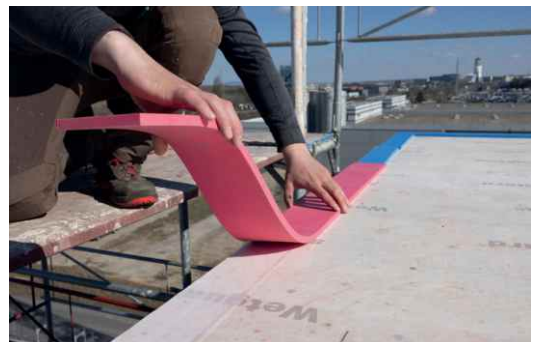
Sylodyn® strips are easy to install. They are prefabricated and are also available as self-adhesive variants.
