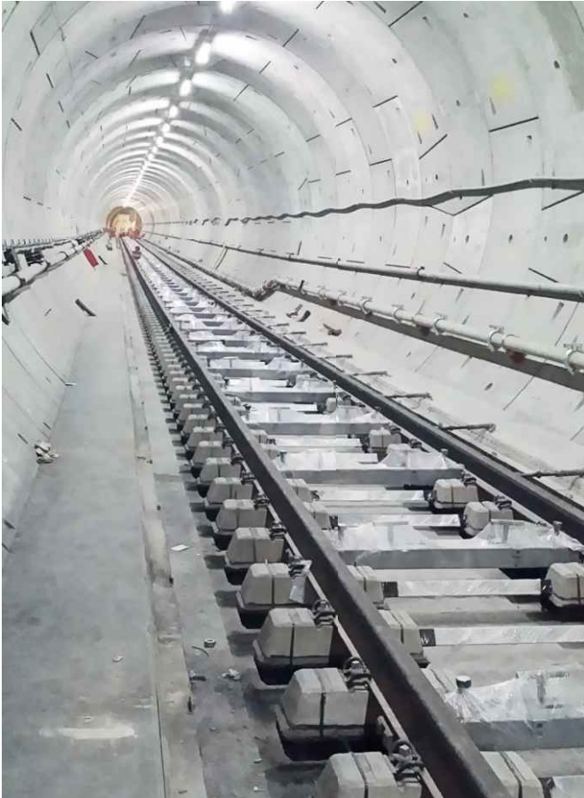
Feste Fahrbahn System in den Tunnels
