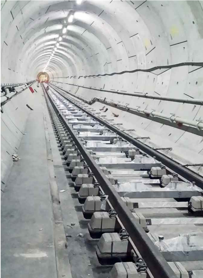
Feste Fahrbahn System in den Tunnels
