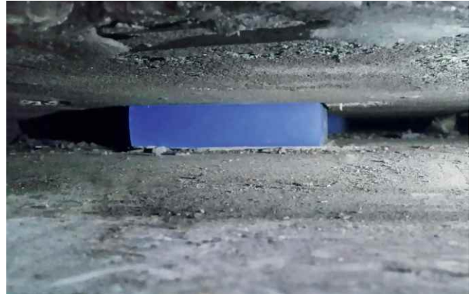
Mass-spring system with Syldyn® discrete bearings
