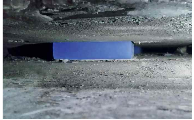
Mass-spring system with Syldyn® discrete bearings
