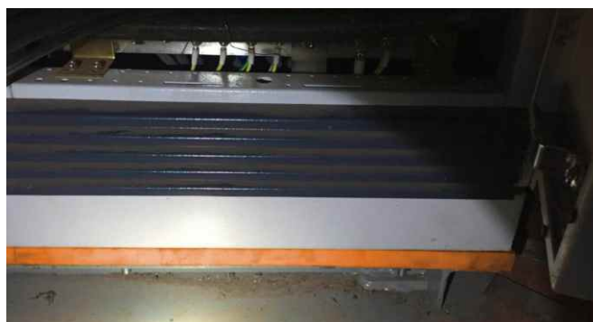
Sylomer® is placed directly under the frame
