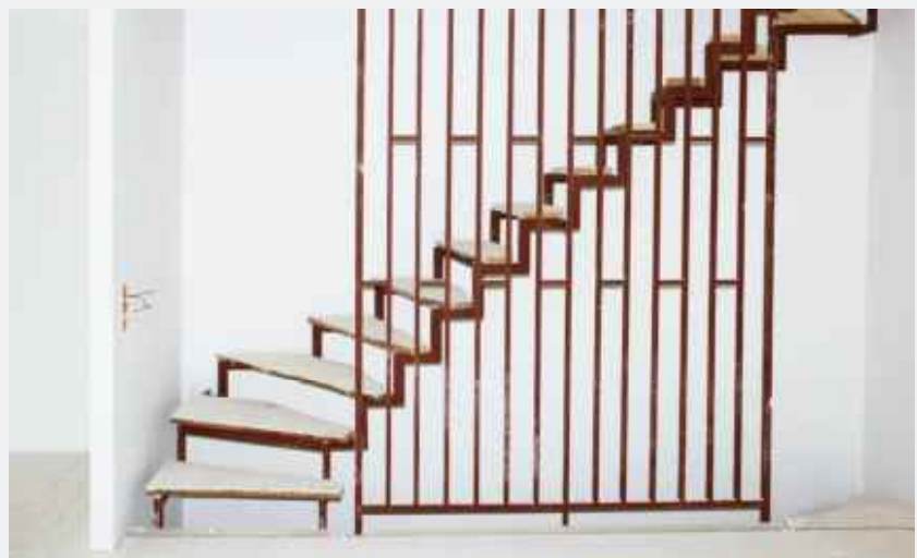
Decoupled harp staircase during construction phase
