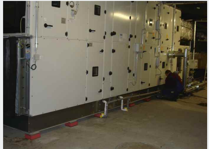
Installation of AC unit on Isotop® SE
