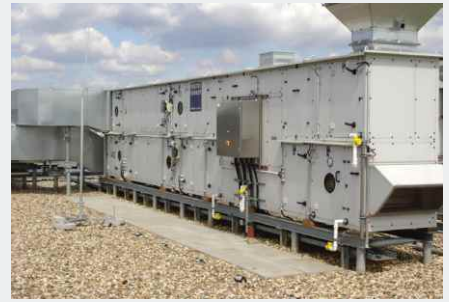
On-roof installation of an AC enclosure
