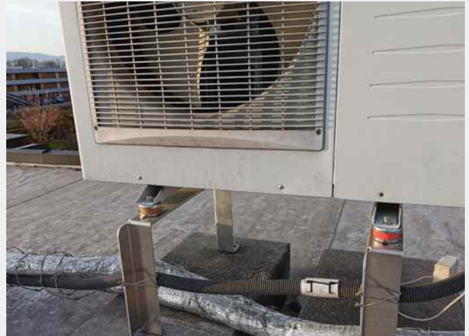
Heat pump bearing with Isotop Compact
