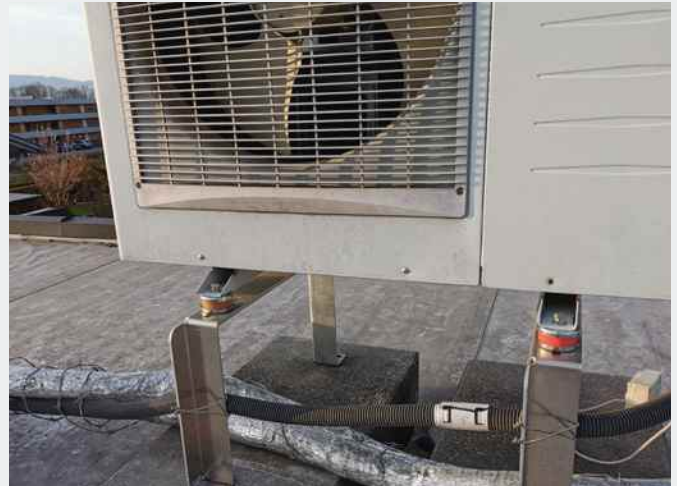
Heat pump bearing with Isotop Compact
