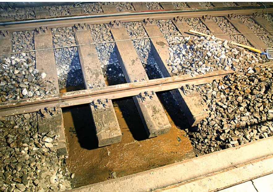
Excavated ballast showing intact mats
