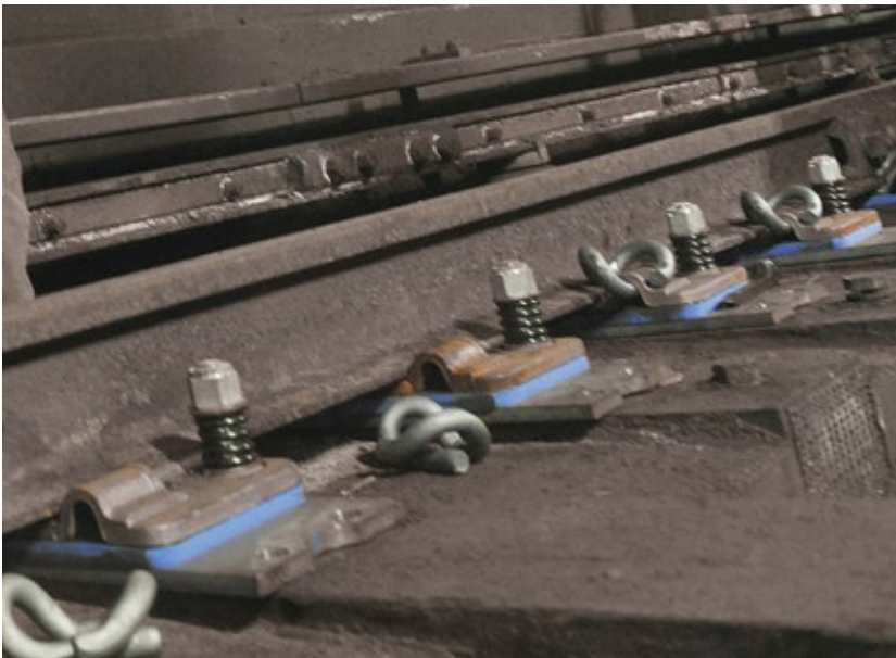
Installation of baseplate pads in the NYC Transit subway system - in use for decades
