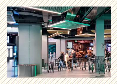
Challenging vibration isolation design: the hotel is attached to the arena using separate, decoupled pairs of pillars – as seen on the left of this photo. The hotel rests on the left side of each pillar, the arena on the right.
