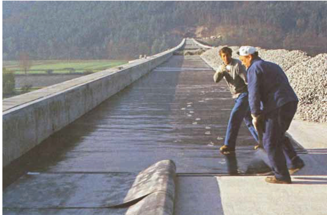
Installation of the Sylomer D 220 ballast mat on the Bartelsgraben bridge in 1987.
